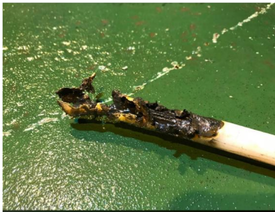
WACS Cable (shunt fault – 2020) in Africa
